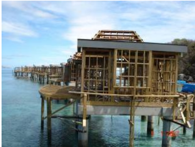
Over-Water Bures taking shape
