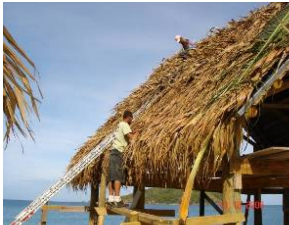
Masima Island Bar roof thatching
